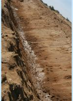
Unlined drainage canals, sandy gravelly soils underlined by poorly permeable bedrock enhanced drainage problems.
